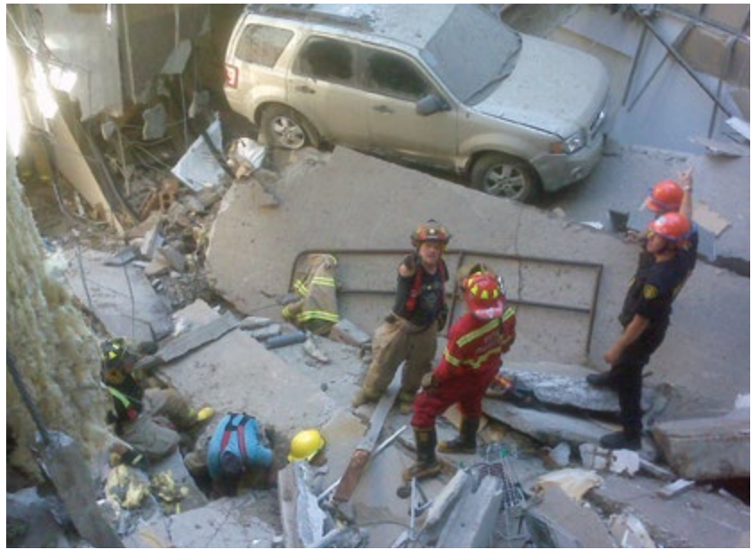
Figure 2.8.1 Firefighters examine voids in the rubble pile
