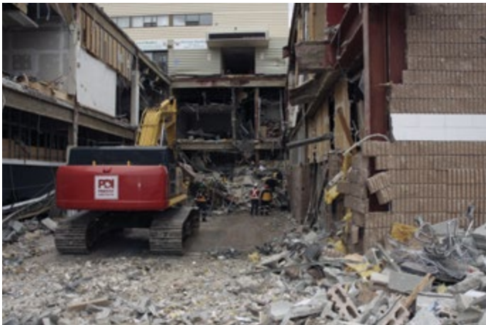
Figure 2.6.9 The Mall interior after the Komatsu 490 cleared out the debris
