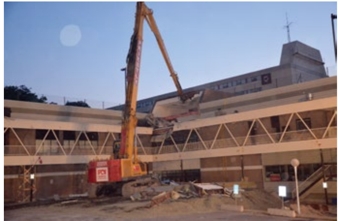
Figure 2.6.7 The penthouse is demolished
