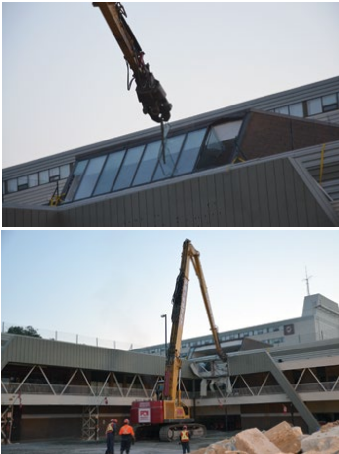
Figure 2.6.6 The Komatsu 850 removing the windows of the penthouse
