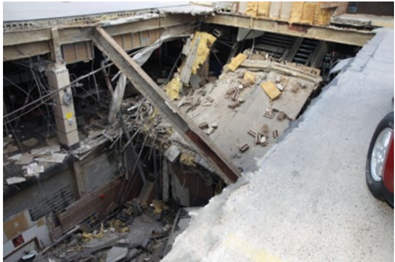
Figure 2.6.1 Concrete slabs and cement blocks laying on top of the slabs
