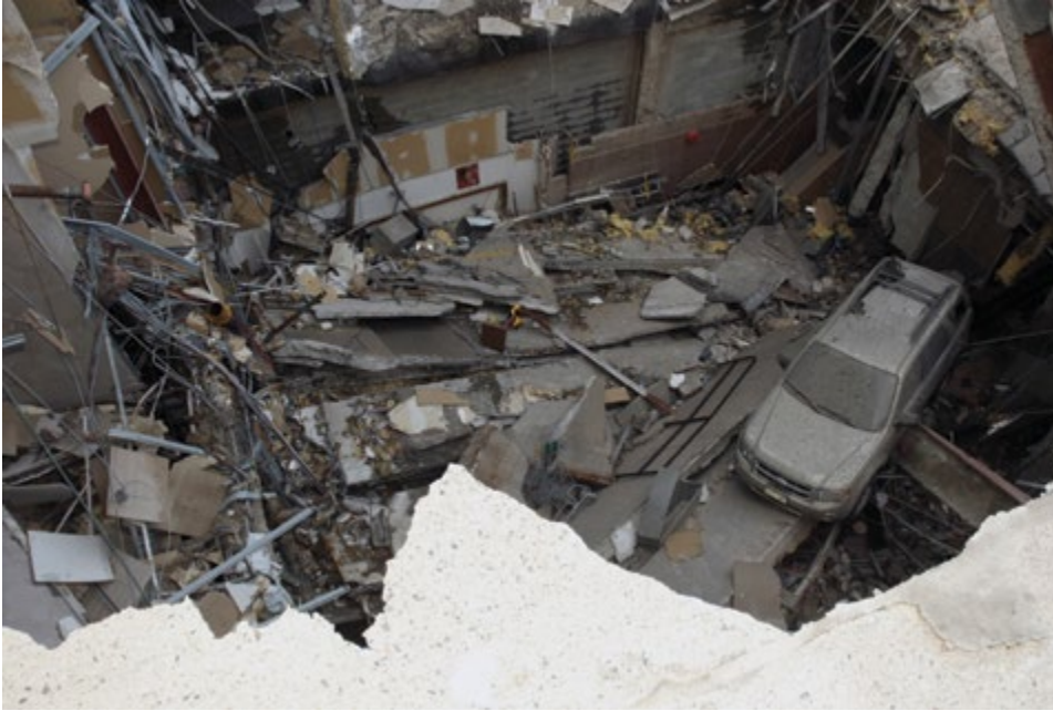
Figure 2.4.5 Ranger gave his positive indication in the area near the railing to the left of the SUV
