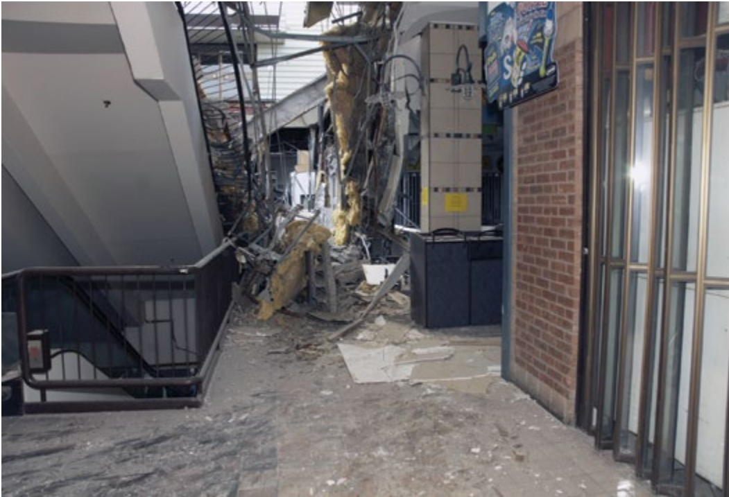
Figure 2.3.4 Second-level concourse facing north toward the kiosk area
